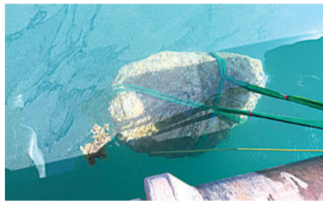
Above: Rock removal
