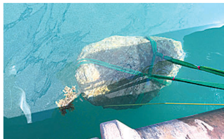
Above: Rock removal
